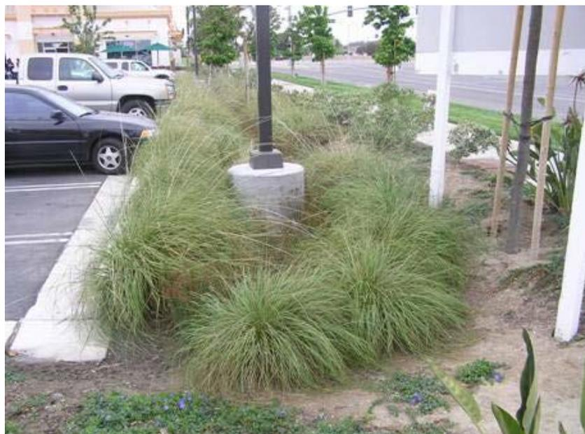
FIGURA 8: ESEMPIO DI TRINCEA FILTRANTE, AIUOLA RIBASSATA CON GRAMINACEE ORNAMENTALI IN CONTESTO FORTEMENTE URBANIZZATO (LOW IMPACT DEVELOPMENT CENTER, INC 2010).
